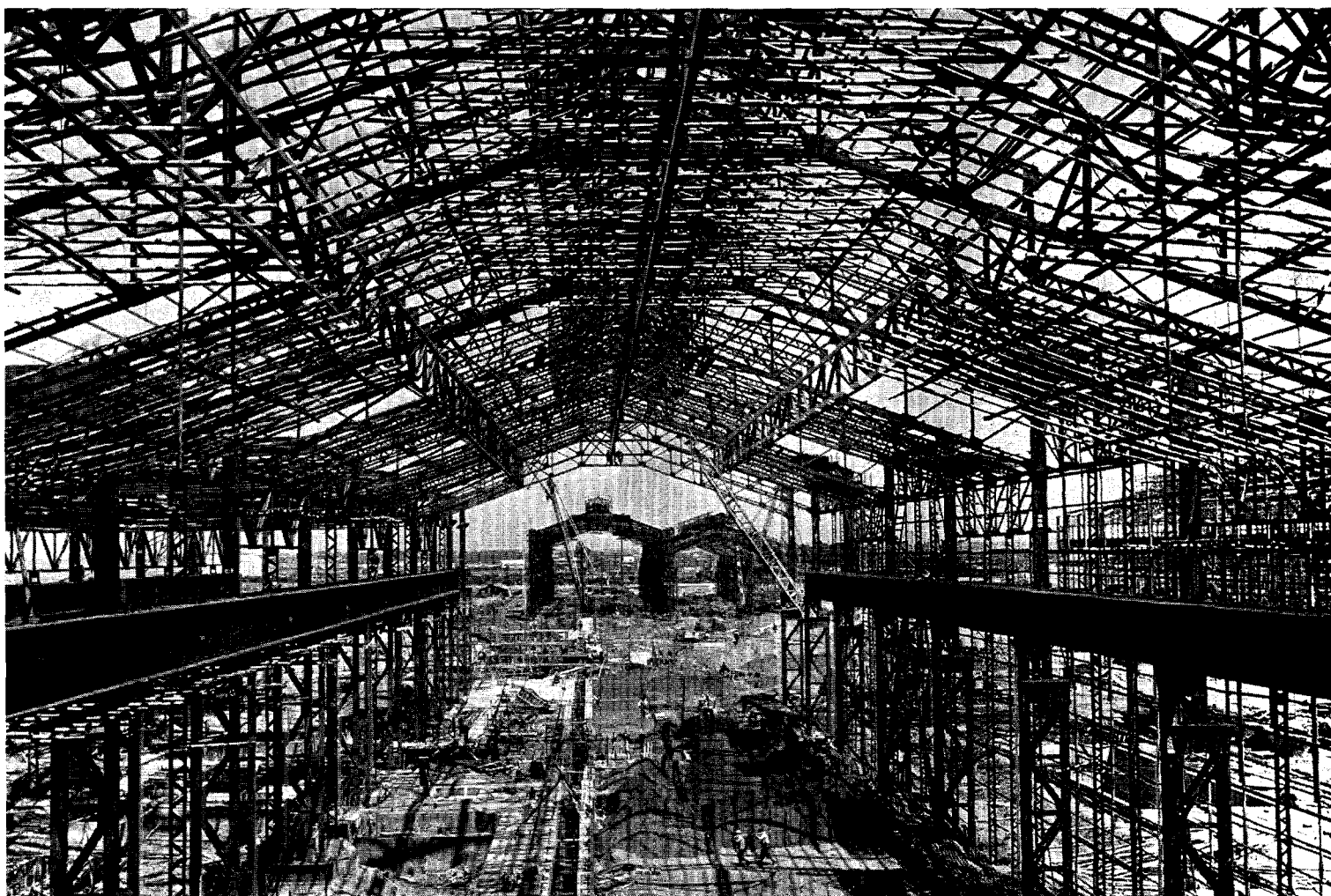
This spider's web of girders shows an early stage of construction of a strip mill, now nearly completed, at the integrated steel plant of the Kawasaki company at Chiba, in central Japan.
