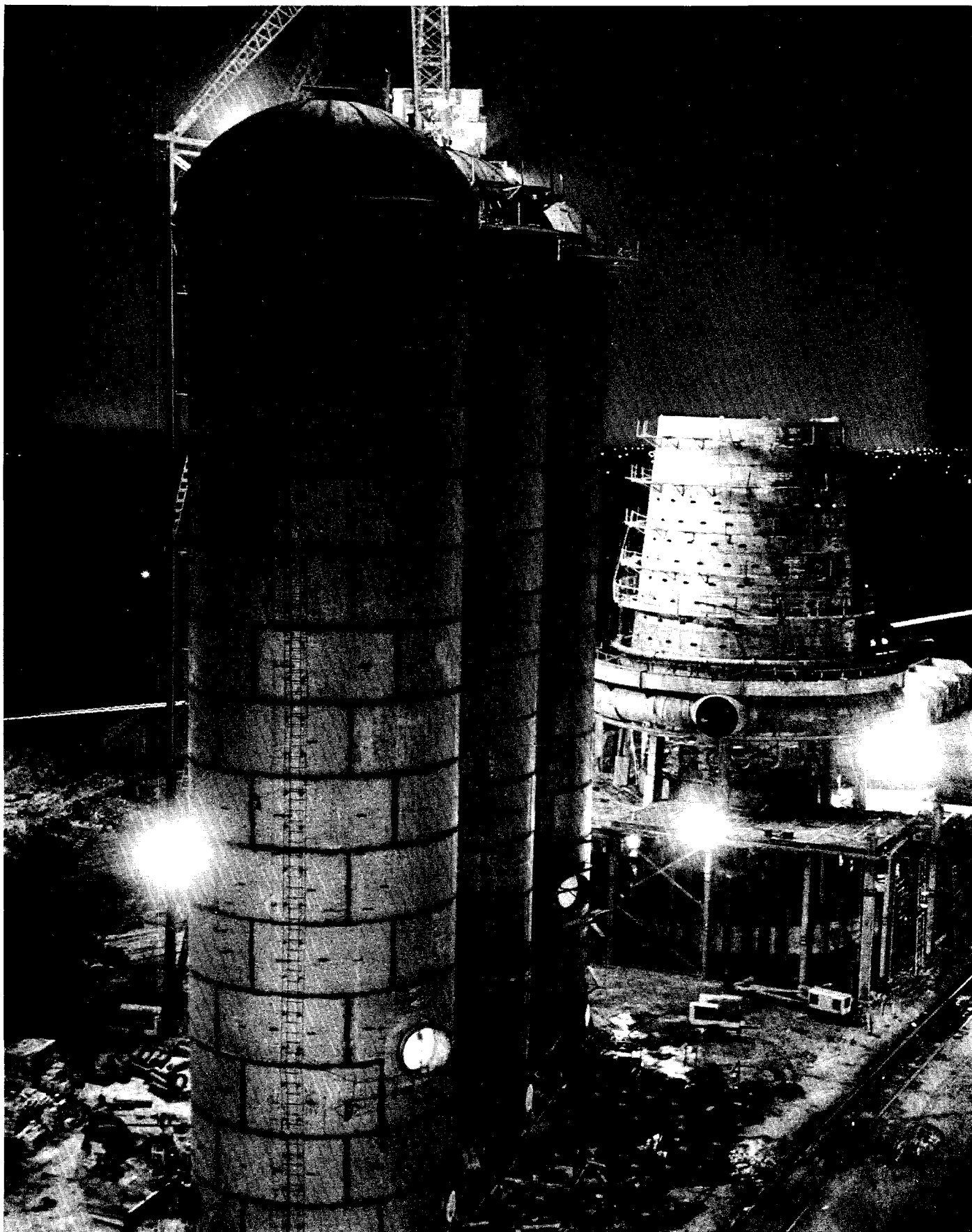
Construction of three hot stoves and a blast furnace — part of the expansion program for the Tata Iron and Steel plant at Jamshedpur — has been pressed forward on a 24-hour basis.
